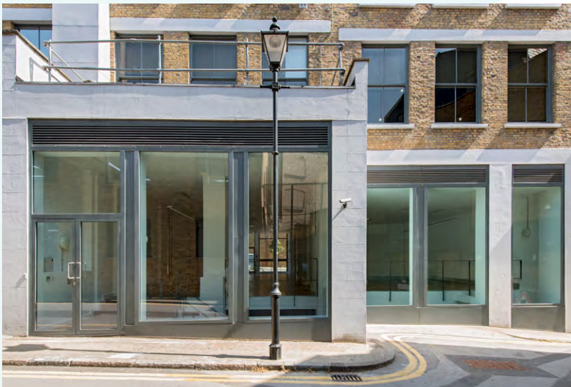
Ground Floor Crawford Passage Entrance
